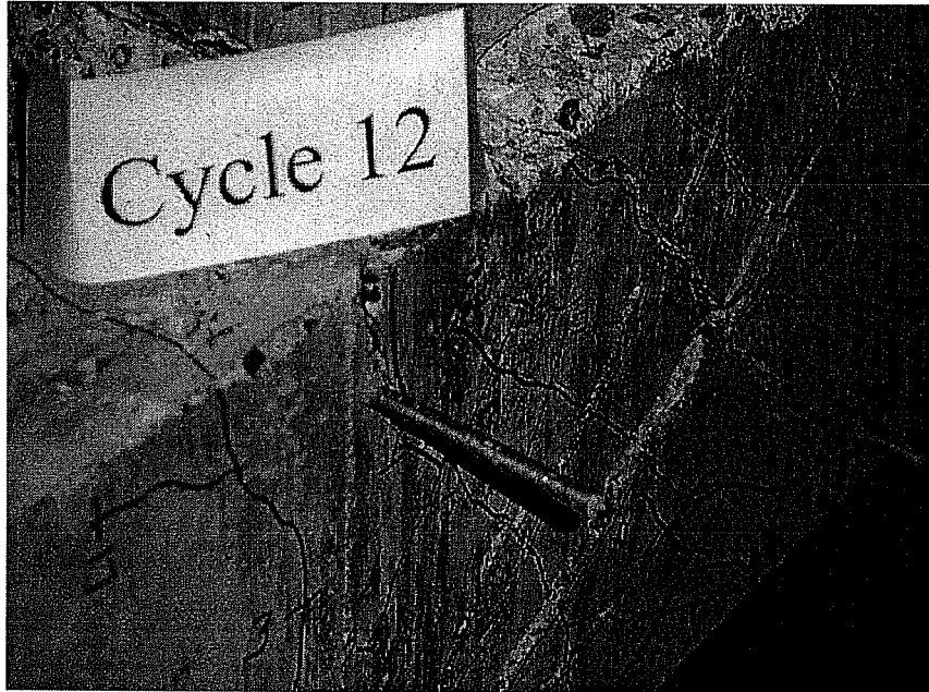
a) Overall View
