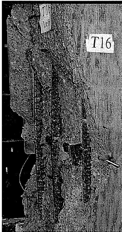
Figure 5.5 Appearance of column bars after failure
