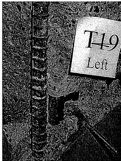
c) Specimen T19 after failure
